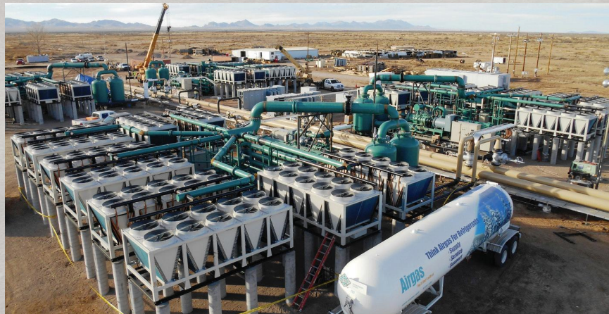
Geothermal energy plants harvest heat stored in the subsurface of the earth to create steam in order to turn turbines producing renewable energy for individual and commercial use.
