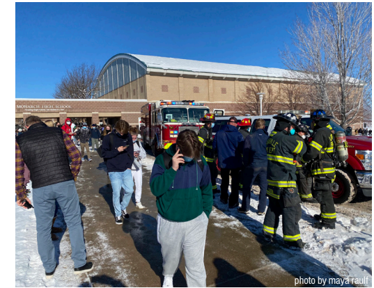
SORRY, WE'RE CLOSED Students evacuate the building before attending any classes due to a chemical leak in the HVAC system on Feb. 3. The district sent out an evacuation notice, which caused many students call their parents for a ride home. "Everyone just all of the sudden kind of left in a panic," Thomas Christopher (9) said.
