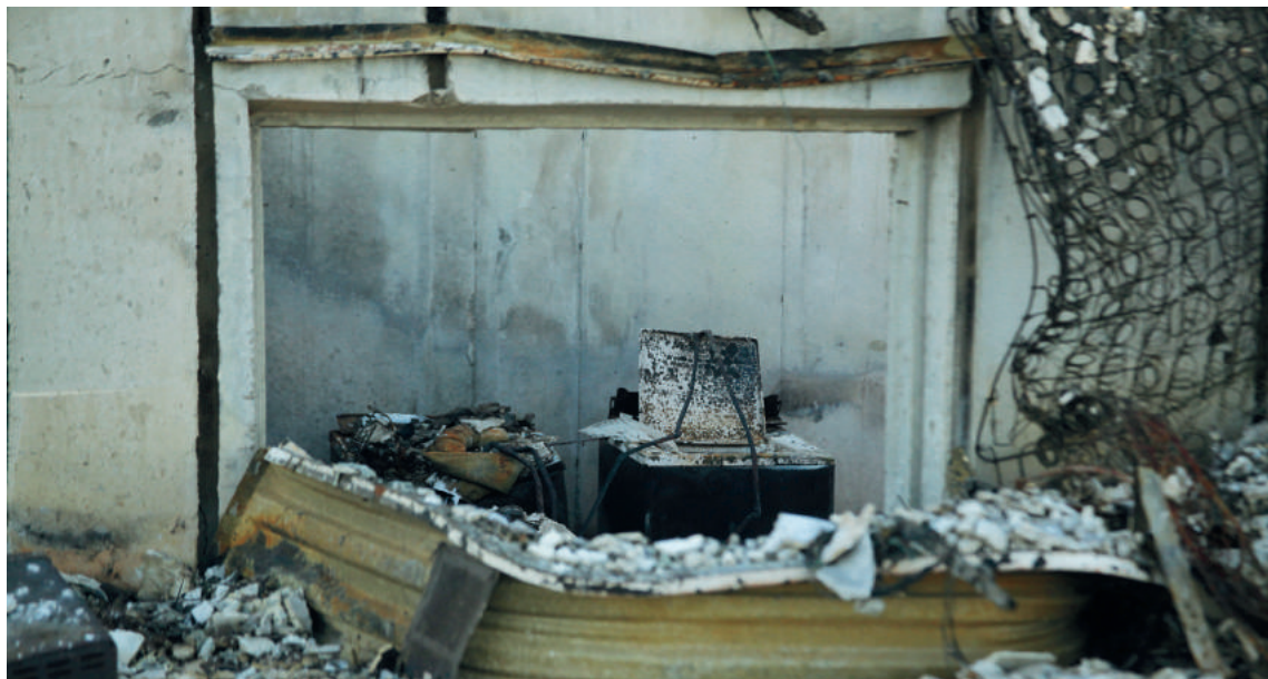
ALL THAT’S LEFT: A burned washer and dryer sit in the basement of a destroyed house in the Sagamore neighborhood in Superior, Colorado. The neighborhood was completely flattened by the Marshall Fire.
